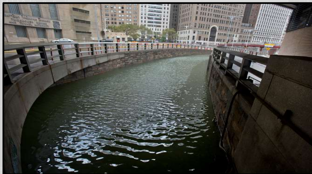
H. L. Carey Tunnel between Manhattan and Brooklyn flooded during Hurricane Sandy, October 2012
